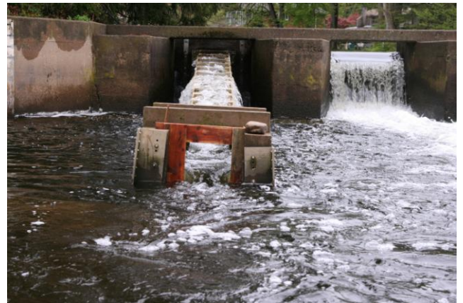
The entrance of the Wood Dam Fishway with a constricting 'footboard' inserted. It throttles down the opening from 24 to 14 inches and has a 24" submerged lip on the bottom. Note there is now a 6" drop in the fishway entrance, creating a stronger flow field issuing out of the fishway entrance, providing better attraction for migrating fish (photo by SH, TNC).
