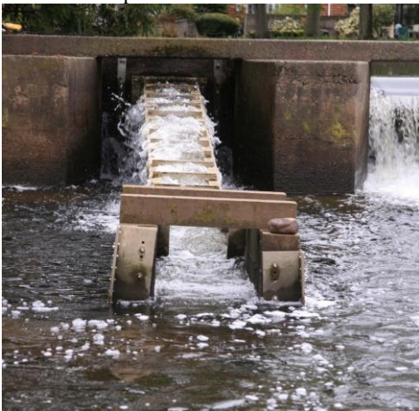
The entrance of the Wood Dam fishway without 'footboard' inserted. Note the lack of strong current issuing out of the fishway. Bubbles from the spillway flow are crossing over in front of the entrance, indicating poor attraction flow (photo by Sally Harold, TNC).
